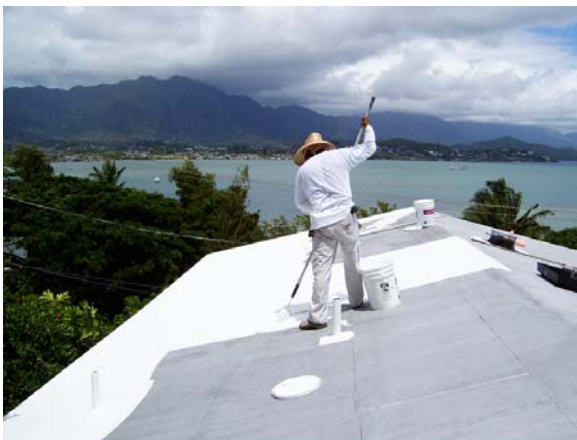
Figure 19: Cool roof installation
